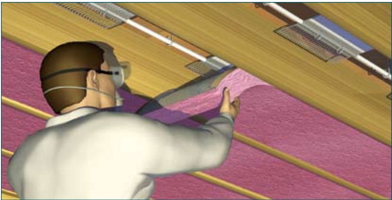
R-12 fiberglass insulation
